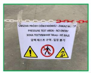
Adequate fencing and marking the danger zone, in which pressure tests will be performed.
