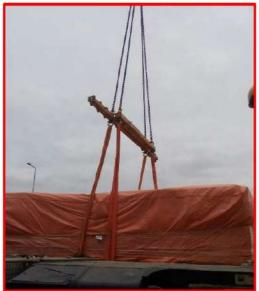
Connecting with each other, tangling in the throat of the hook and layering the slings as well as using materials and devices not intended for this type of work for lifting loads is prohibited. Hand hoists (chain, rope) are not slings and cannot be used for this purpose.
