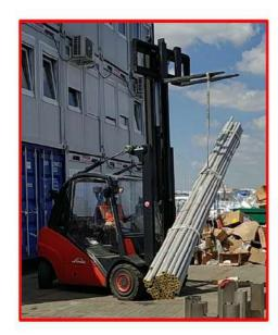
Hitching the load to the forks of motorized trolleys and other devices of this type, eg Manitou, is allowed only and exclusively with the use of dedicated transport traverses. The use of lines, belts or slings and other materials not intended for this purpose is prohibited.
