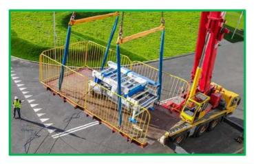
The load transported by the transport platform must be secured against moving while being lifted. Disconnecting the cargo securing devices is possible only after the platform is docked to the anchoring points in the target building.
