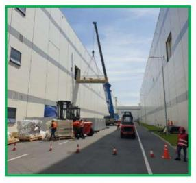
The securing of the target area where the pickup is carried out must be mandatory prior to commencing any work. It is forbidden to leave the opening in the facade of the building without protection with permanent barriers locked with a "key" and a tarpaulin.
