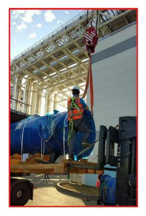
An employee is not allowed to stand on the load, over a load or under a load that is suspended or lifted.
