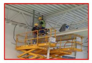
The work area should be properly enclosed and workers should use the required personal protective equipment when operating mobile platforms and have the necessary fire extinguishing agents in the workplace.
